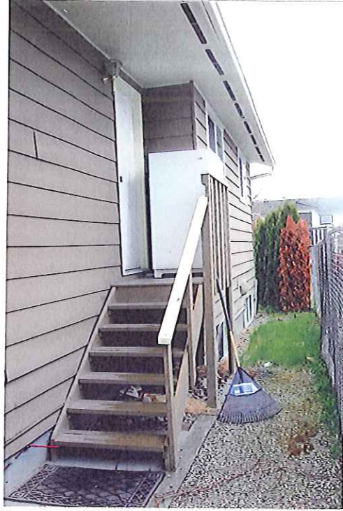
east side suite entrance
